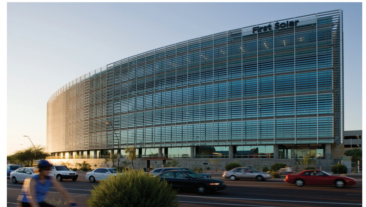
First Solar is a LEED Gold building. Its most striking sustainability feature is the computer controlled exterior louvers used for sun control.
